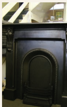
1850s-'60s Cast iron combination fireplace. This surround is very common in Ireland and can be found in the main living room of mid-range terrace houses and in the bedrooms of grander houses. Value: €450-€900 depending on size
